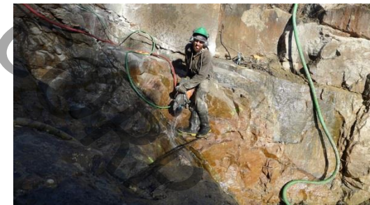
(Sampling Rod production pit – 2015)
